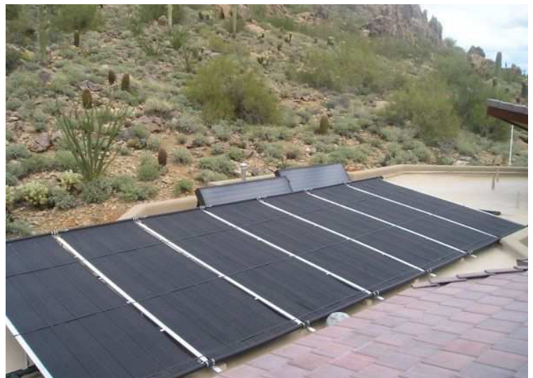
(below) Solar panels for both pool and domestic hot water.
